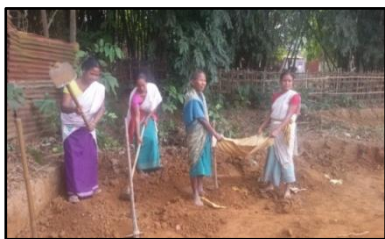
Figure 1: Women Labourers Digging Land
